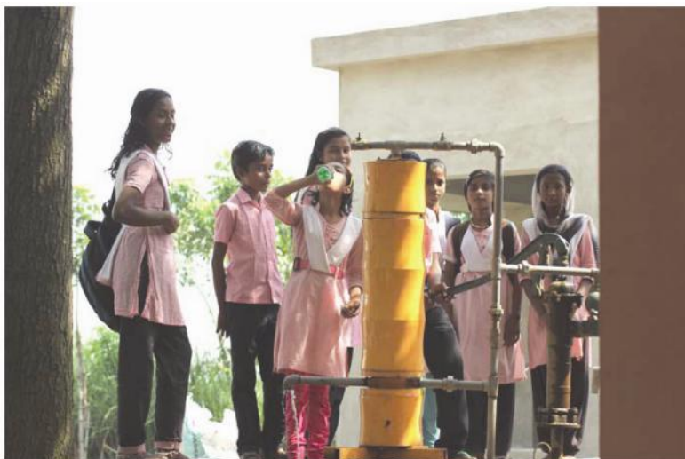
Figure 1. Scene from a school in Nadia district, West Bengal. Children are drinking water from a filter which removes iron and arsenic selectively, attached to a hand pump. The technology was developed by IIT Madras and was commercialized by an IIT Madras incubated company with the support of the district administration and the Government of West Bengal.
