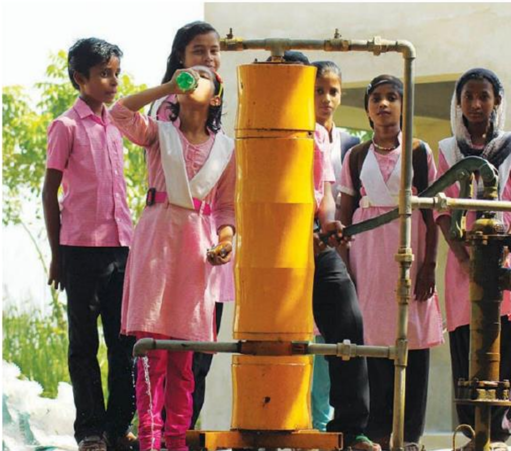
A water purification unit using nanomaterials connected to a handpump © Indian Institute of Technology, Madras
